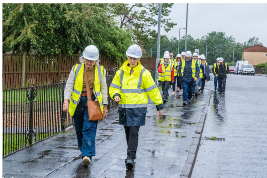
Commissioners visiting a large-scale social housing retrofit site in Coatbridge
