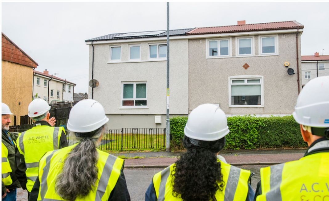
Commissioners visiting a large-scale social housing retrofit site in Coatbridge
