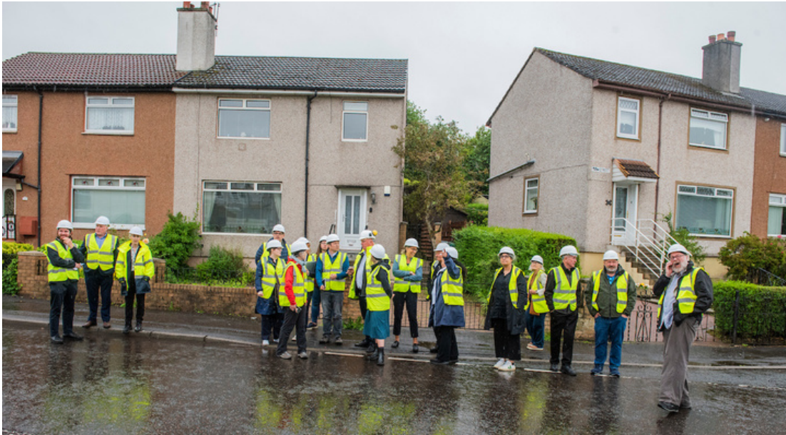
Commissioners visiting a large-scale social housing retrofit site in Coatbridge
